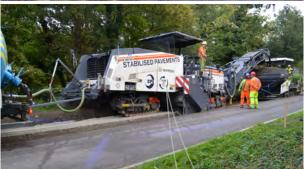
The recently completed £3.4m scheme on the A1066 near Thetford saw a section of road surface replaced between Thetford and Diss. Routine monitoring showed a rapid deterioration of the surface following the hot summers of 2018 and 2019 which left the busy route very uneven in places.
