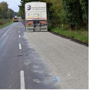
Since the mixed material is placed through the paver levels are set and, following compaction, falls ensure cambers remove water from the carriageway. In this case 2.5% from the centre line to the side of the road.
